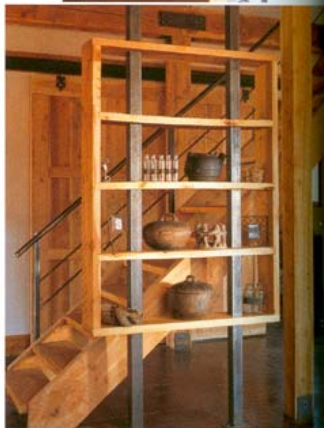
●●● SHELF SCREEN. The shelving unit bridges the gap between the rough-hewn timber-frame structure and the slab stair, partially screening the living room from the hallway.
